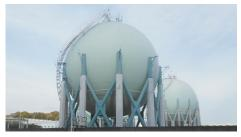
Brace retrofitting for a spherical tank
